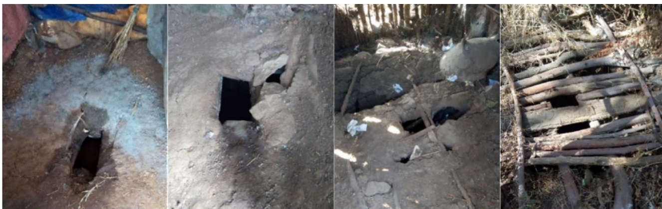
Figure 2 Traditional dry pit latrines usually do not sustainably segregate excreta from human contact.
